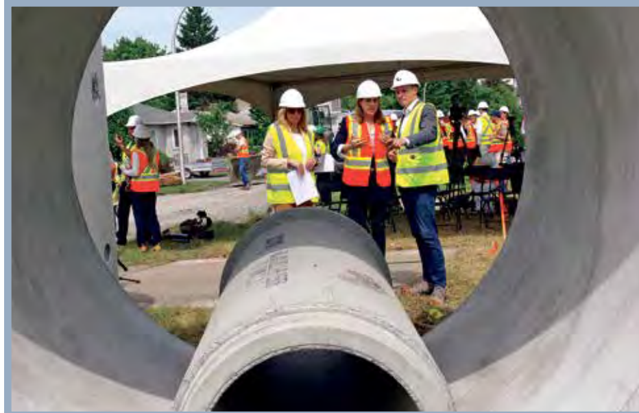
From the left, Vimont MNA Valérie Schmaltz, Quebec Environment and Fight Against Climate Change Minister Pascale Déry and Laval mayor Stéphane Boyer go over some points with supersize rainwater drain pipes ready to be buried at a work site in Vimont last Monday morning. (Photo: Martin C. Barry, Laval News)
