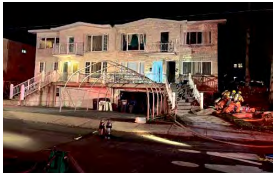
The fire-damaged home on 66th Ave. in eastern Chomedey. (Photo: Association des pompiers de Laval)
