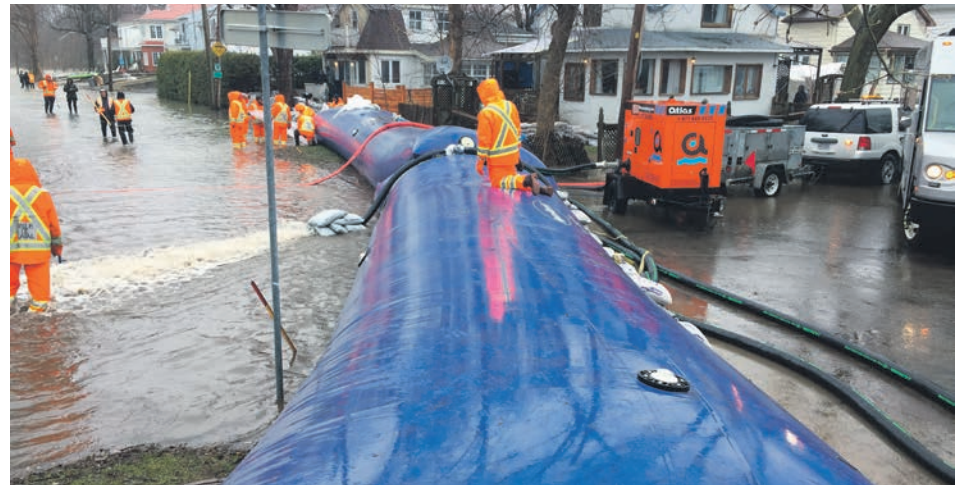
This Aqua-Barrier set up at the corner of 30th and 17th streets in Laval-Ouest was useful in keeping the surging waters of the Rivière des Mille Îles in their place. PHOTO: Martin C. Barry (TLN-NEWSFIRST ARCHIVES APRIL 2019)
